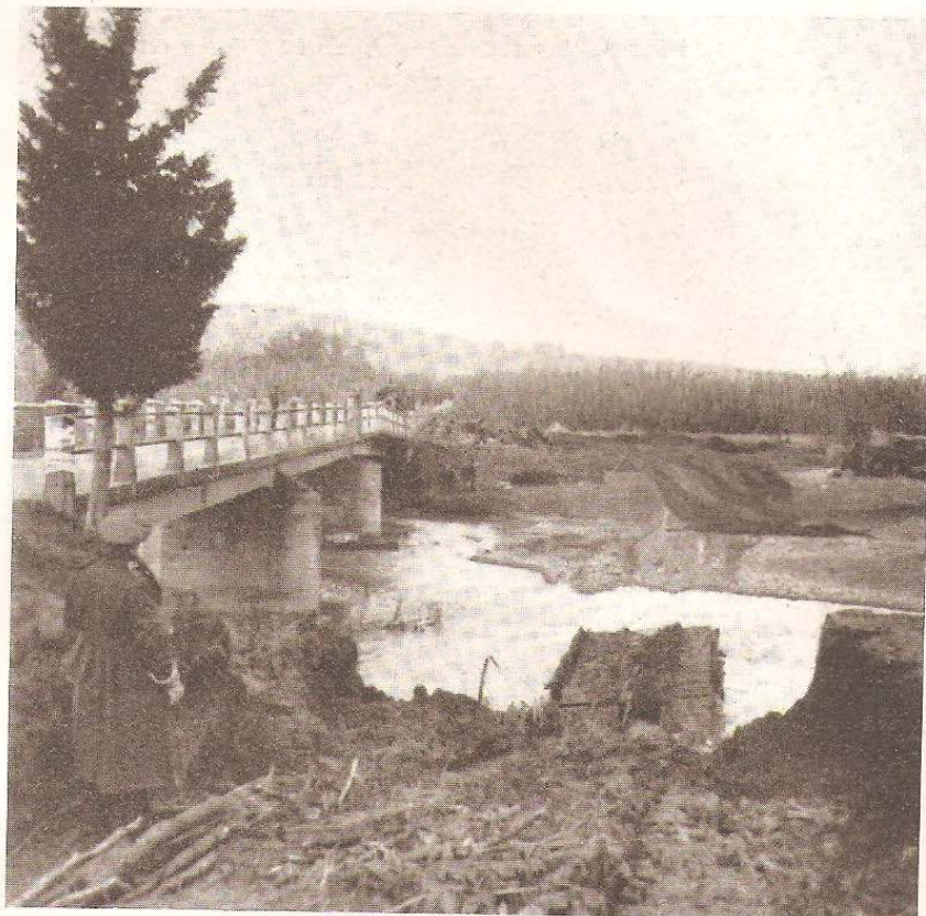
The bridge at Terre del Sale
